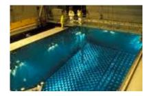
"The storage pool at Vermont Yankee Nuclear Power Station was originally licensed to hold 600 spent fuel assemblies. There are now 2,935 assemblies in the pool, or 932 metric tons of radioactive waste."
