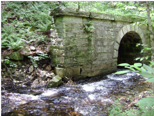
RR Bridge below Bennett Brook Road
