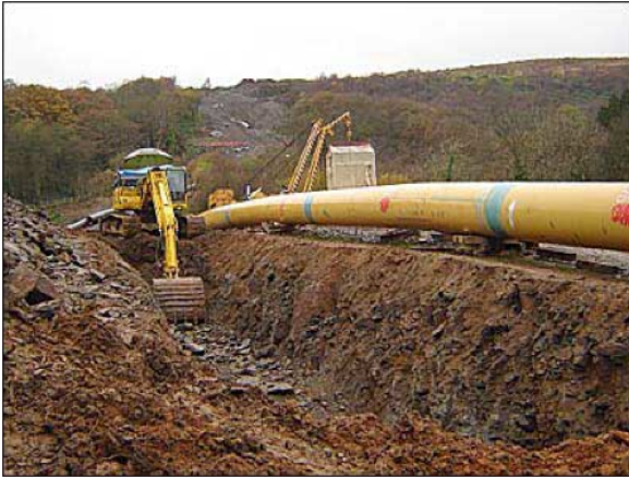
Pipeline would be 30-36" in diameter and buried 3 feet deep
